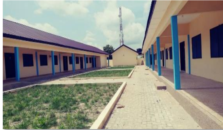
Single-storey Dormitory Block at Nkoranza Technical Institute, BA
