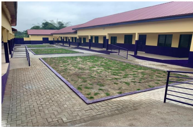
Single-storey Dormitory Block at Kwabeng Anglican SHTS, E/R
