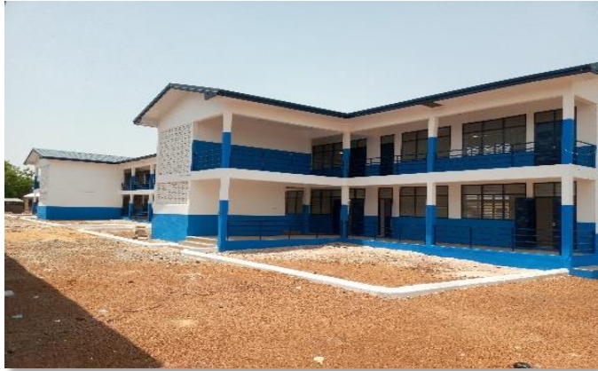
12-unit Classroom Block at Savelugu Senior High School, N/R
