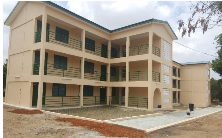
3-storey 18-unit Classroom Block at Odorgonno Senior High School, G/R
